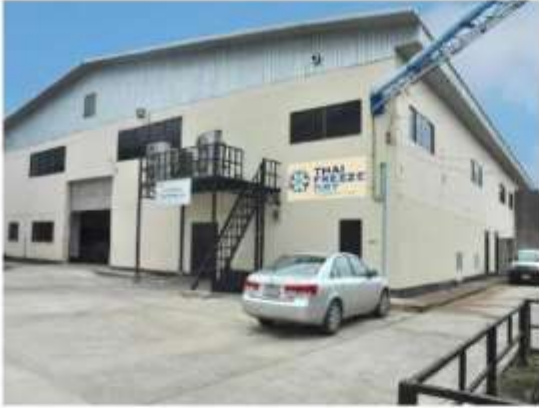
TFD Factory Premises
